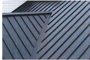
METAL STANDING SEAM ROOF
